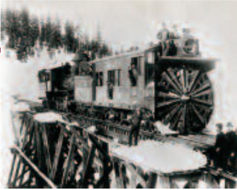
**1884** A patented valve regulates steam in a rotary snowplow designed and built by Leslie that rescues trains otherwise stranded in snow drifts and blizzards in the isolated winter terrain of the northern United States and Canada, where rail is commonly the only reliable mode of transportation. So durable, several of these original 1800 era snowplows with Leslie valves are still in use over 100 years later.
