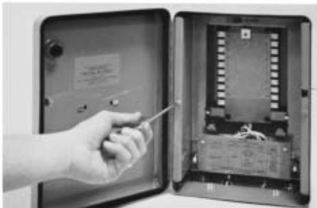
5. Assemble the control and module and install the unit into the modernization adapter. Tighten the chassis retainer.
