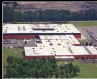
CONWAY, SC Steel Foundry and Manufacturing Plant
