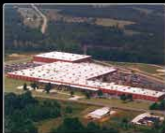
PAGELAND, SC Final Assembly and Distribution Center
