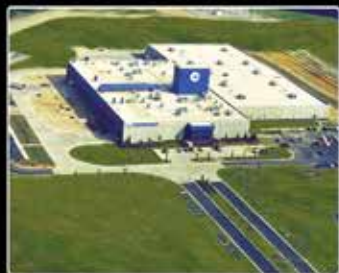
PAGELAND, SC Bronze Foundry and Manufacturing Plant
