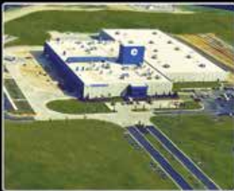
PAGELAND, SC Bronze Foundry and Manufacturing Plant
