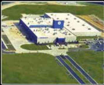
PAGELAND, SC Bronze Foundry and Manufacturing Plant
